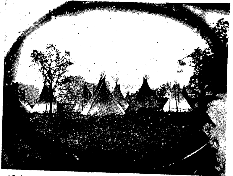
1854 -- The original neighborhood. This land eventually became Bridge Square (see lower photo on next page). MHS photo.
