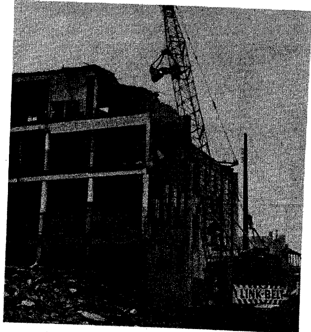
Demolition along E. Hennepin. Photo: N.P.
